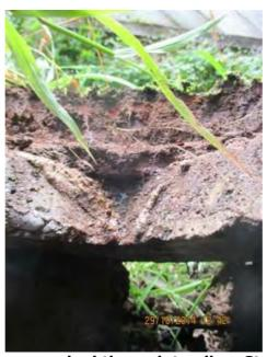
Figure 1: Opening smashed through to allow Storm water entry
